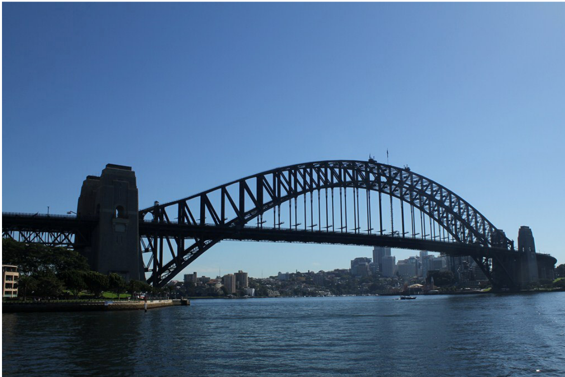
Foto 16: Harbour Bridge Sydney
