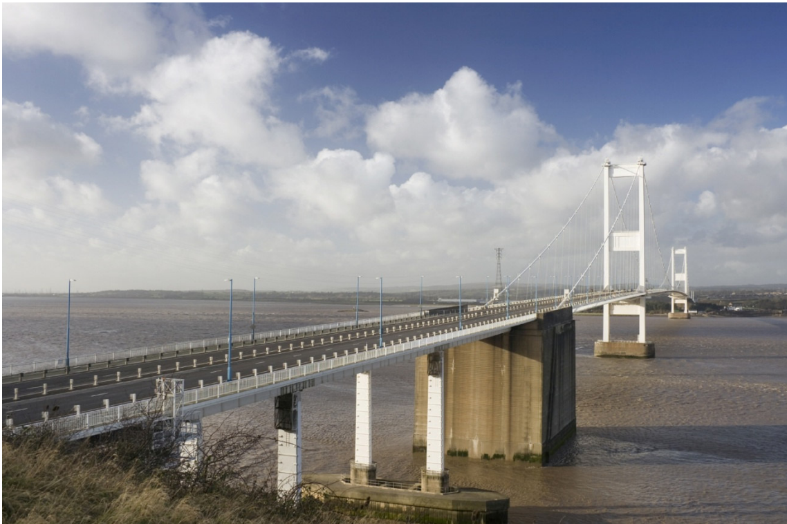
Foto 28: Severn-Brücke in England
